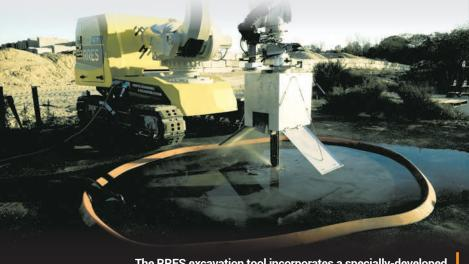
The RRES excavation tool incorporates a specially-developed chainsaw designed to cut through reinforced concrete
