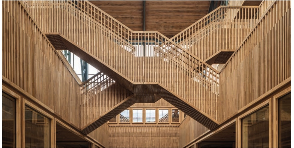
Above: The upper mezzanine floors are cantilevered out from the core and a special joint had to be developed to support them
